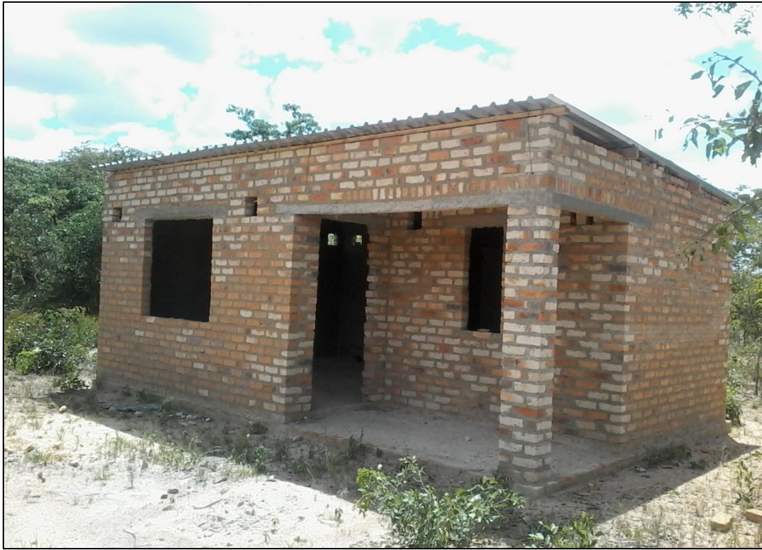
Picture 8: A house being built at Mbuya Kamuzanga's farm by her son
